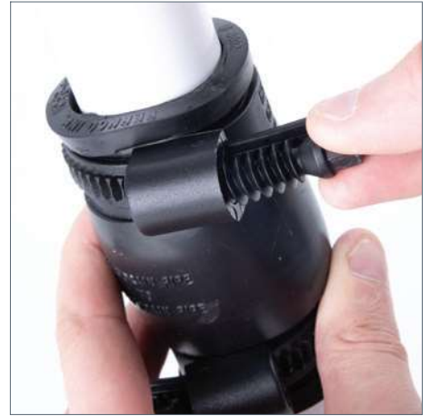
Insert Screw into Housing
