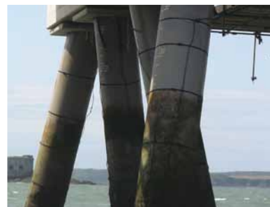
Corrosion Protection - Anode Attachment
